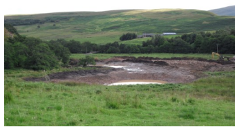
Fire pond under construction
